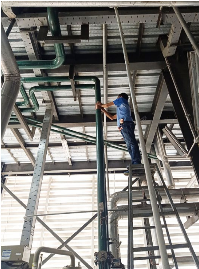
Installing Vulcan S25 for the new chiller.
