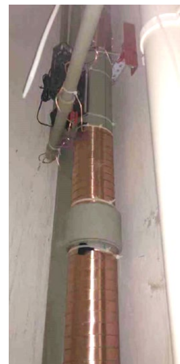
Vulcan S50 is installed on the main water pipe
