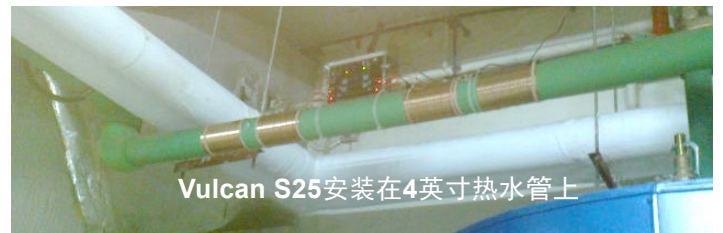
Vulcan S25安装在4英寸冷水管上
