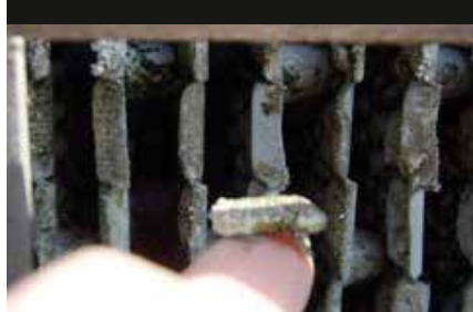
Silica could not be removed by the high pressure water gun, but can be peeled off with a nail.
