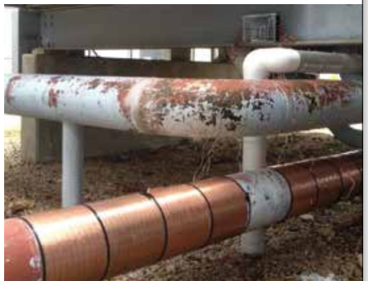
Vulcan S250 installed on a 10 inch diameter line that feeds twin cooling towers (CT-1 and CT-2)
