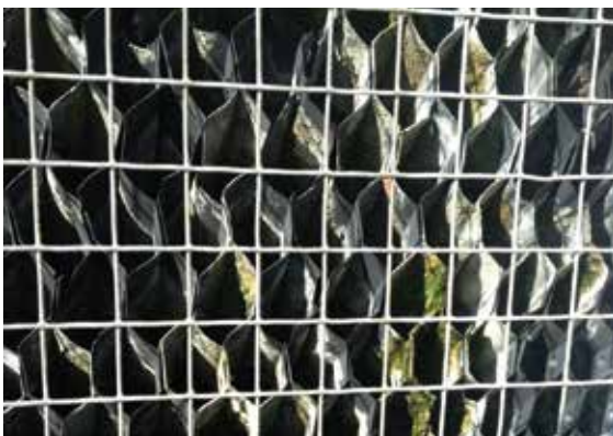
The photo above was taken of CT-1 about 3 weeks after the Vulcan was installed.
