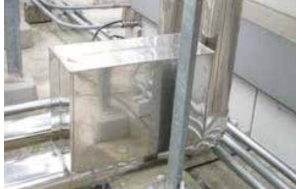
Vulcan S25 was installed on the makeup water pipe for the cooling towers A, B and C.
