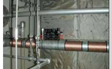
Vulcan S25 was installed on the circulating water pipe for the cooling towers C.
