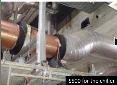
Impulse bands covered by pipe insulation
