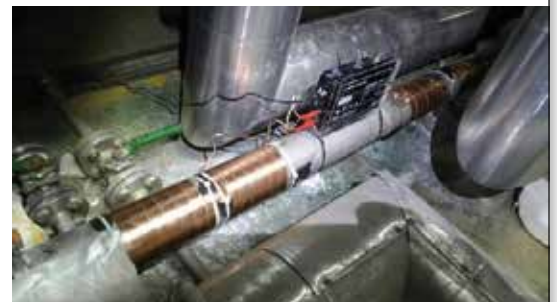
Vulcan S25 installed at Toray Industries
